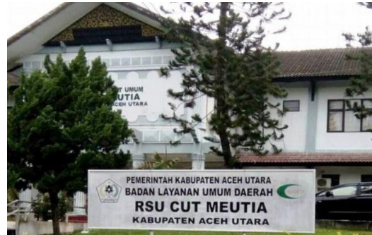
Public Hospital in Lhokseumawe
